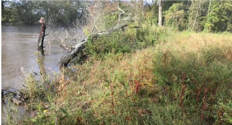
French Broad River Bank Stabilization
