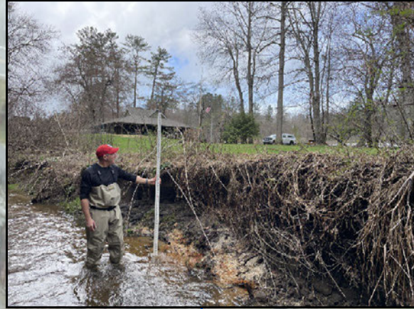
Site 14 (230 linear feet, left bank) Estimated erosion rate: 7.0 tons/year
