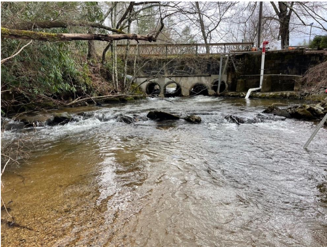
Figure 6. Cardinal Road Bridge Crossing.
