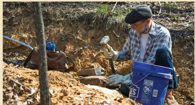
Stefan Israel crushes rocks for gravel to fill in log steps. Photos by Pat Barcas.
