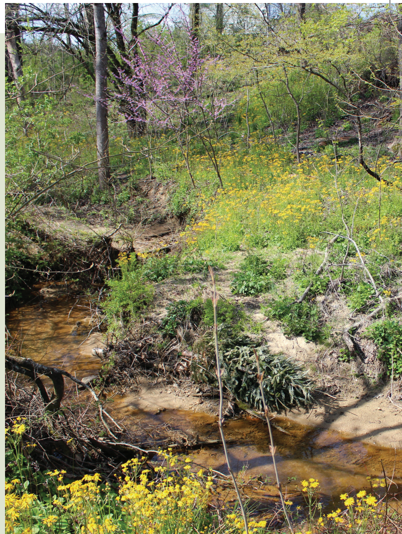
At our Hendersonville office, Tom Fanslow, our land protection director, recycled a Christmas tree by securing it to an eroding stream bank with rebar. The Christmas tree's branches help stabilize the bank, allowing live stakes positioned among the branches to grow into trees.
